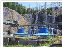
The two generators are each capable of producing up to 225 MW of power.
