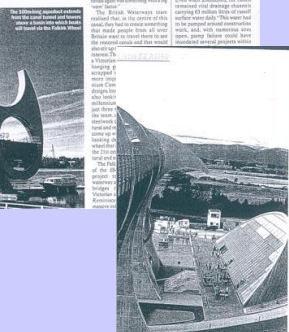
The Falkirk Wheel is a rotating boat lift. It is the lynchpin of a 1.10km waterway across central Scotland. It is the most dramatic element in the canal system.
