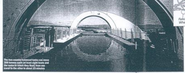
The Falkirk Wheel is a rotating boat lift. It is the lynchpin of a 1.10km waterway across central Scotland. It is the most dramatic element in the canal system.
